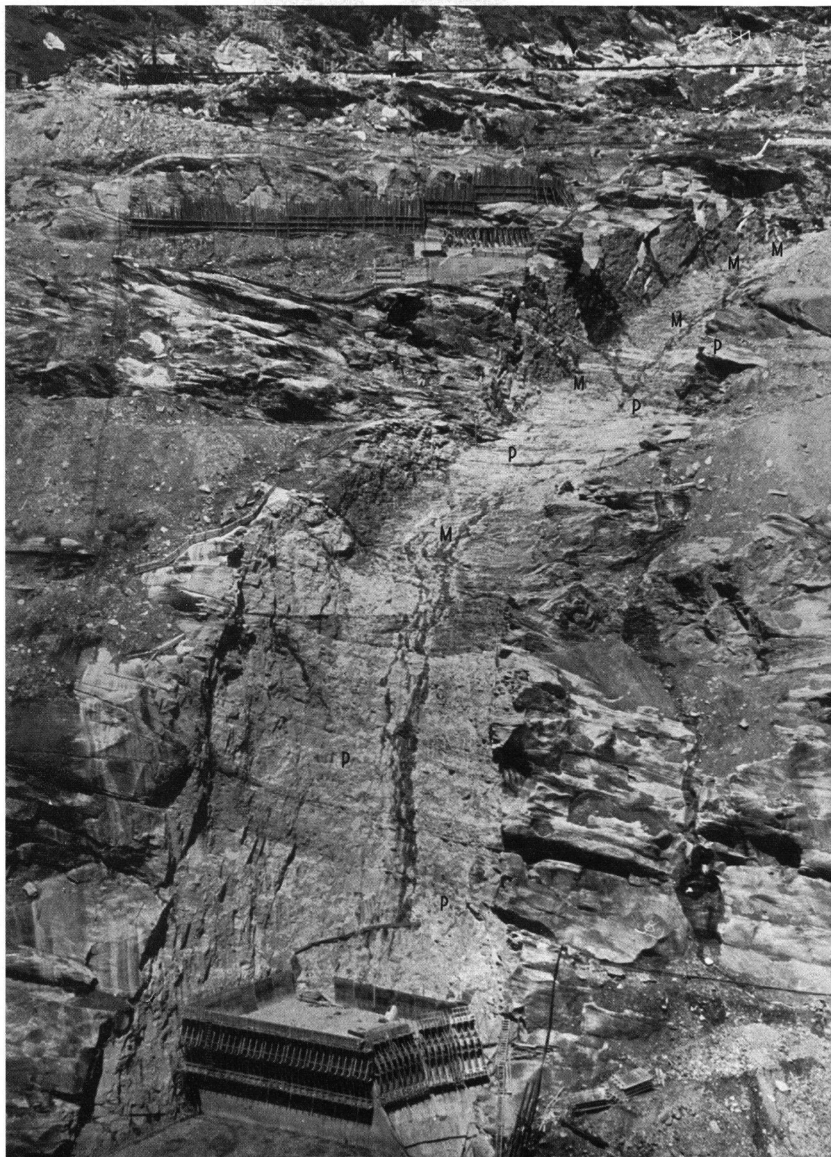
Fig. 8. Northern part of the trough of the Zervreila dam, as exposed in august 1956. P = phengite-gneisses; M = mica-schists.
